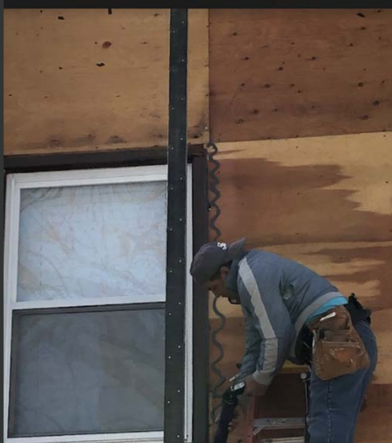
Liquid flashing application at window jamb
